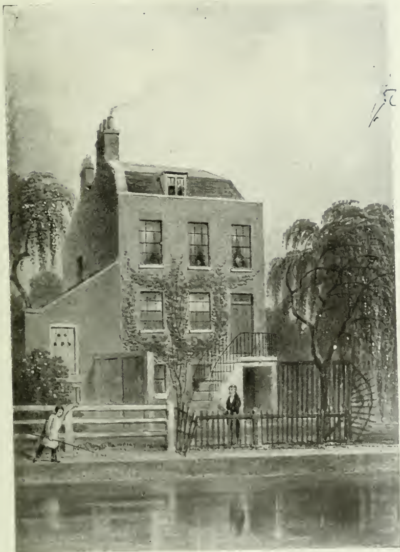
COLEBROOKE COTTAGE, AND THE NEW RIVER. LAMB'S HOUSE AT ISLINGTON
